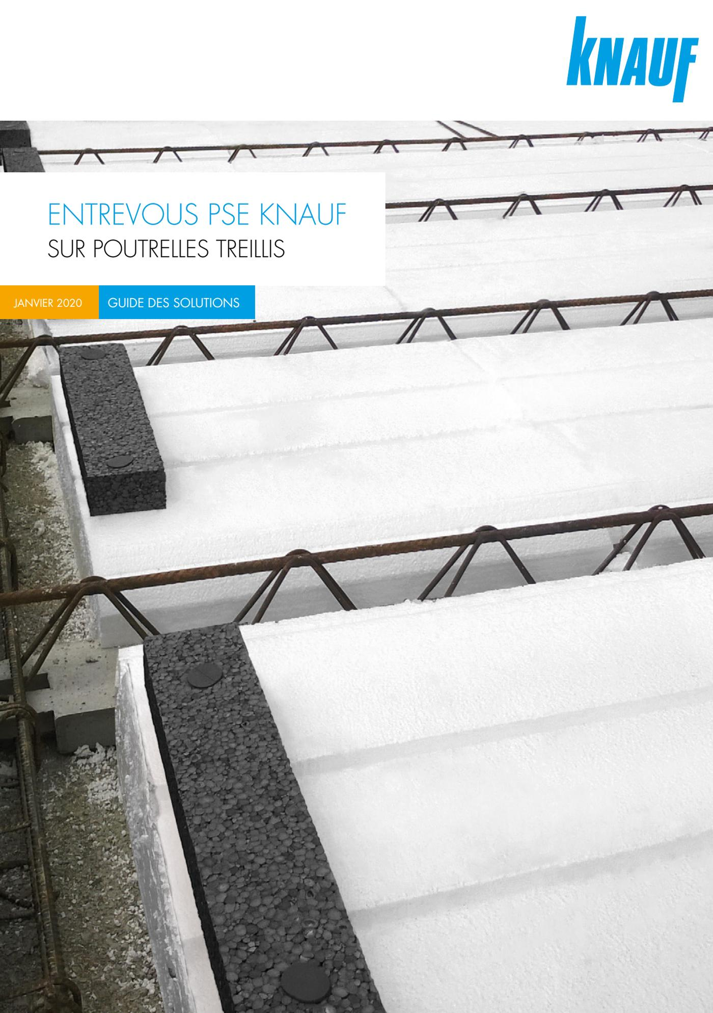
The background of the entire page is a photograph of a construction site. It shows a series of parallel steel reinforcement bars (rebar) supported by metal brackets. Large, white, rectangular panels of expanded polystyrene (EPS) are placed between the rebar. The panels are being prepared for a concrete pour. The perspective is from a low angle, looking down the length of the structure.
